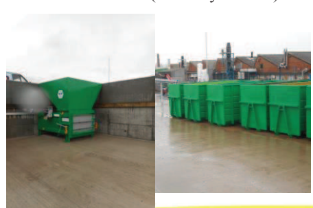
Household Waste (service yard side)
