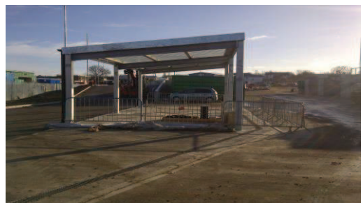
Canopy area (Oil, Paint etc.)
